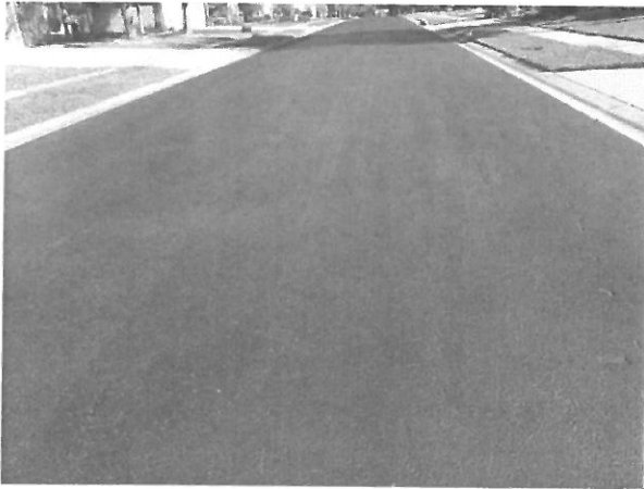
Asphalt pavement at Safe Harbor Lane
