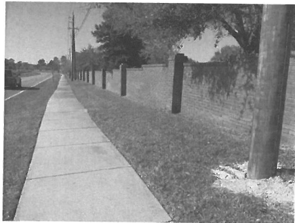
Masonry perimeter wall
