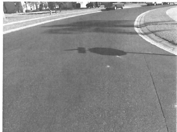
Asphalt pavement at Tidal Pool Cove
