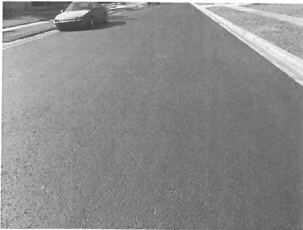
Asphalt pavement at Night Breeze Lane
