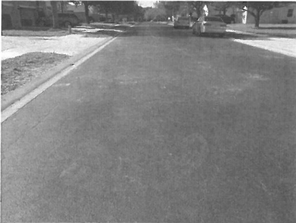
Asphalt pavement at Reagan Trail
