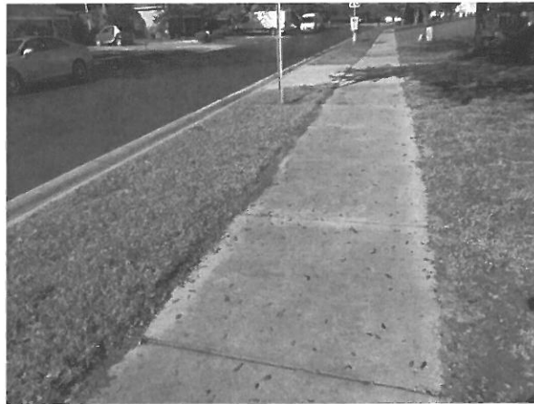
Typical concrete sidewalk
