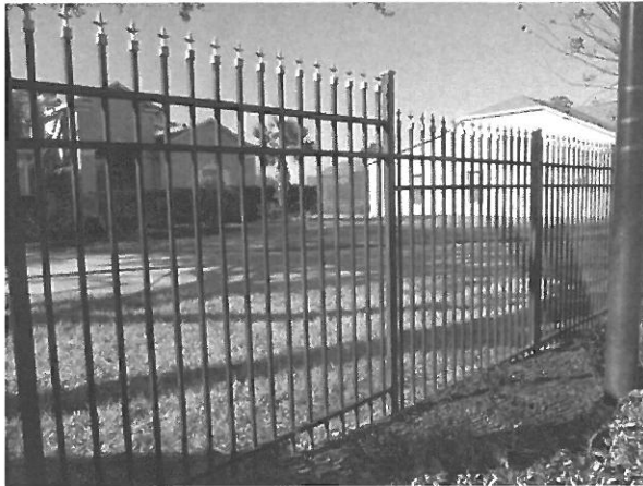
Typical aluminum fence at entrance
